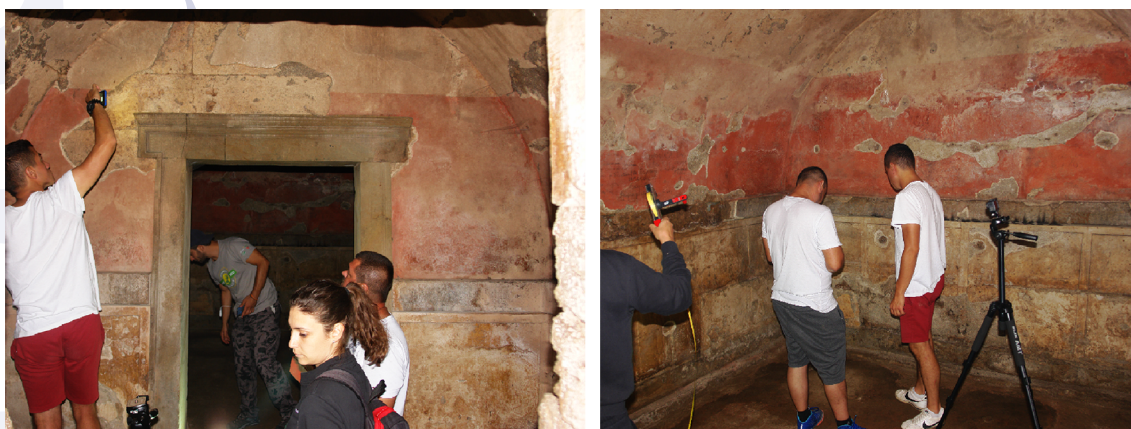
Figure 2. The survey and documentation of the Ohrid tomb (photo I. Malezanov, D. Angjelkovski).
